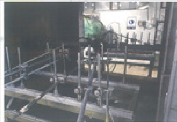
Setting test Thermocouples
