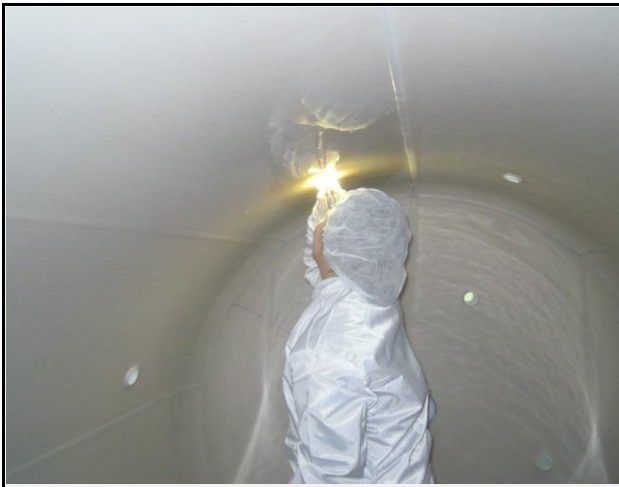
LINING INSPECTION - VISUAL
